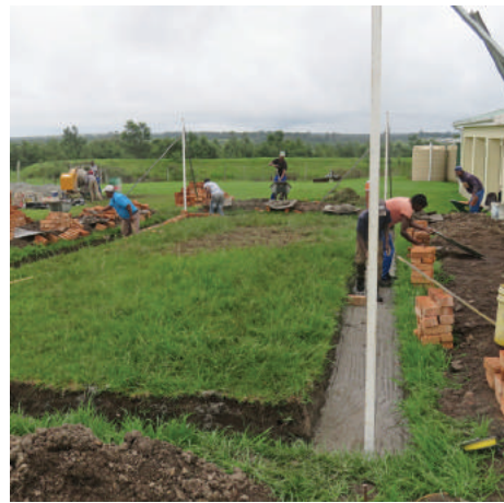
The foundation for the new laundry building
